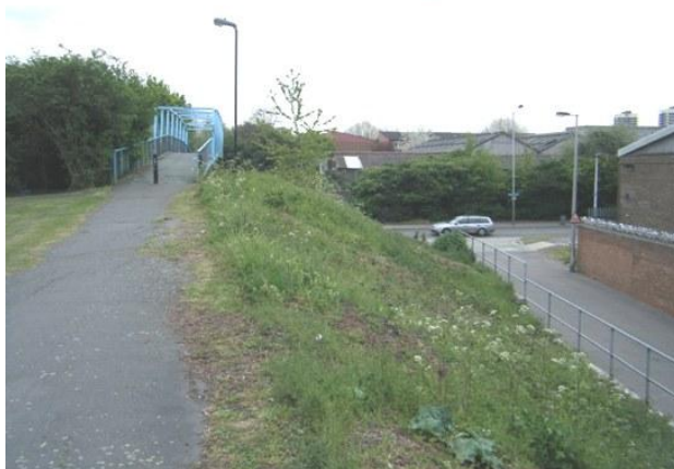
Figure 5.8: Current Footbridge Across Surrey Canal Rd
