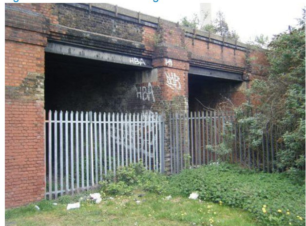
Figure 5.7: Network Rail Bridge . Arches for ELL
