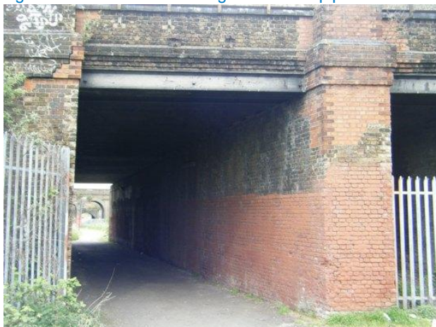
Figure 5.6: Network Rail Bridge . Arch for pipes
