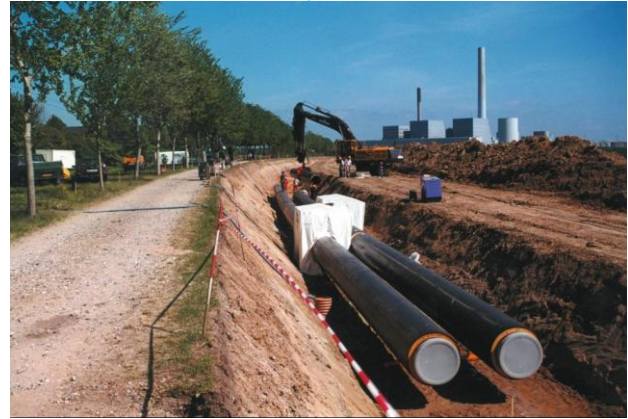
Figure 5.2: Installation of large diameter pipe
